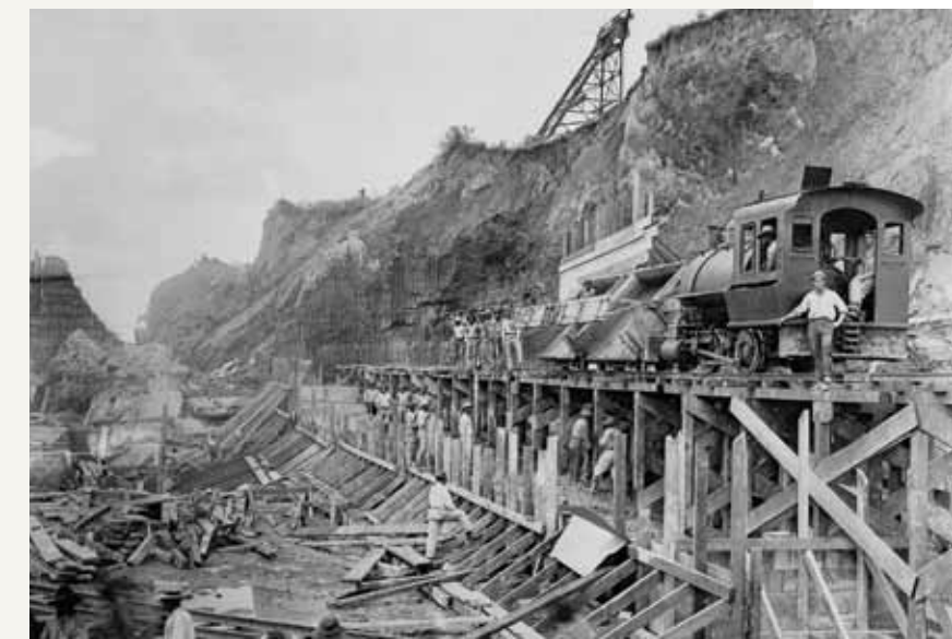
RIGHT: The most taxing daily labor was the excavation of the Culebra Cut. Each day workers moved miles of construction track and filled the spoil trains that ran in and out of the Cut. Landslides often buried workers and equipment.
